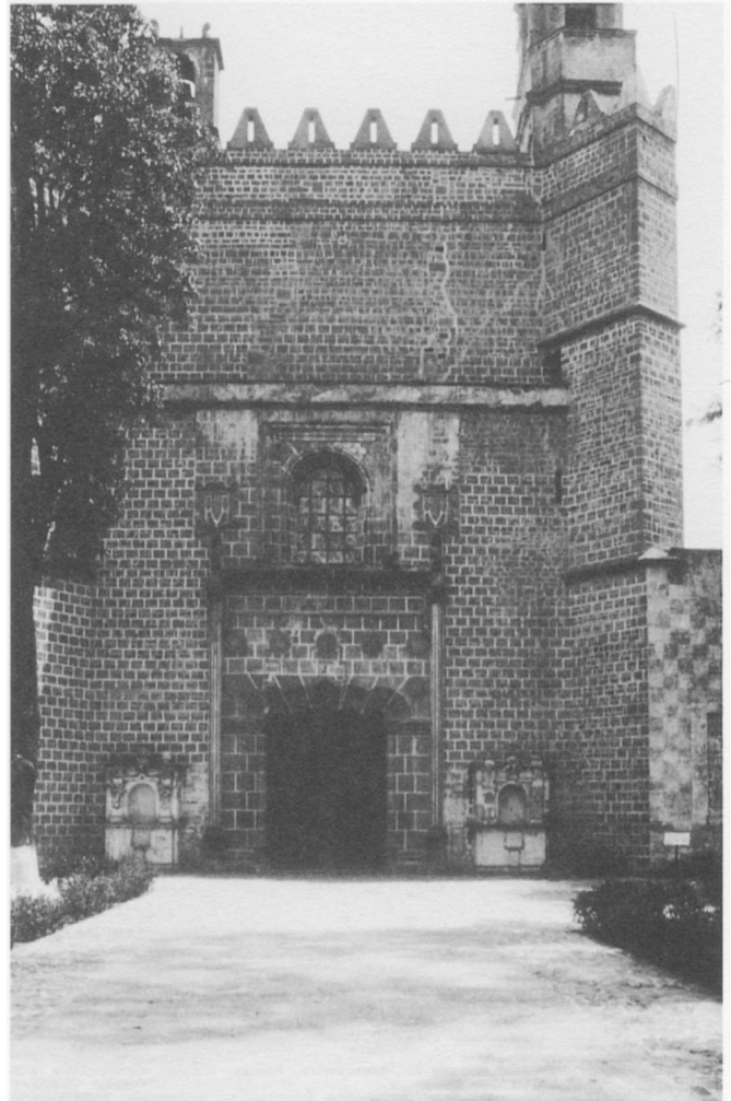
Figure 3. Juan de Alameda, Franciscan Monastery of San Miguel, main facade of church, Huejotzingo, Mexico.
